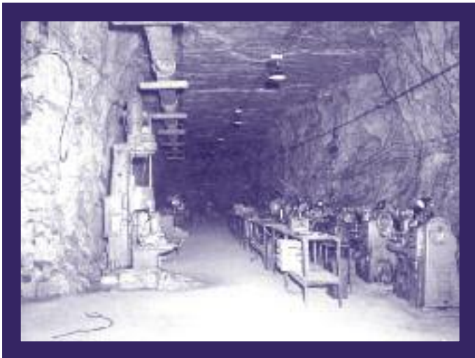
View into one of the production galleries after the concentration camp prisoners had been withdrawn, September 1944
