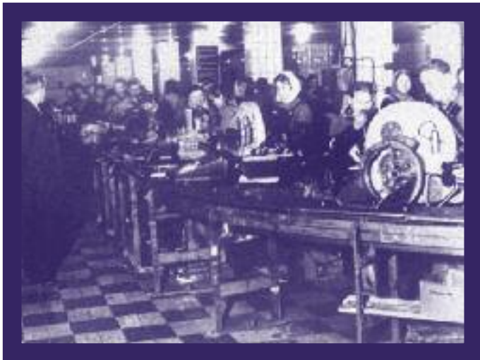
The continuous engine assembly line in the washroom of the mechanical workshop, 1944
