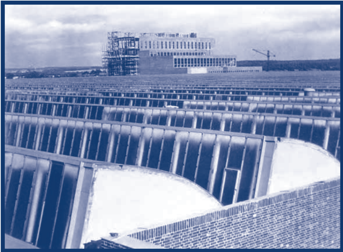
View of the shed roofs of the factory halls and the power station, 1939
