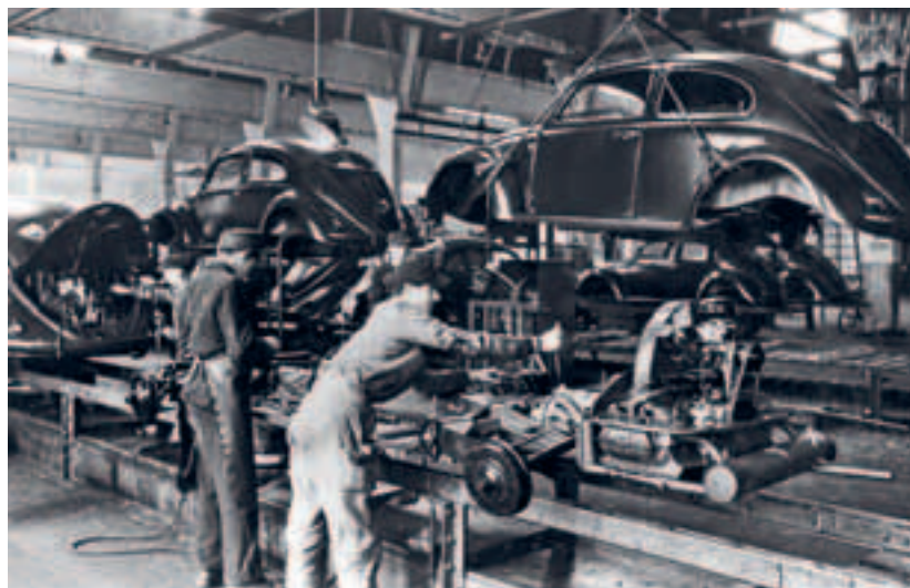
ASSEMBLING LINE IN WOLFSBURG
